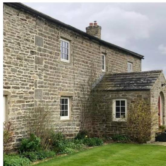
Figure 3: Example of older stone wall dwelling
