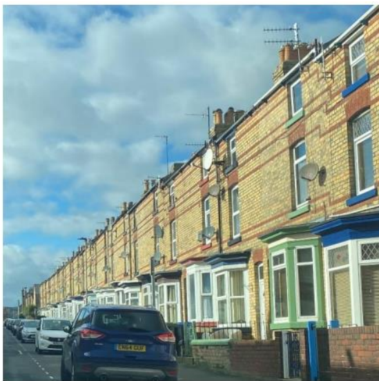
Figure 2: Example of Victorian terraces
